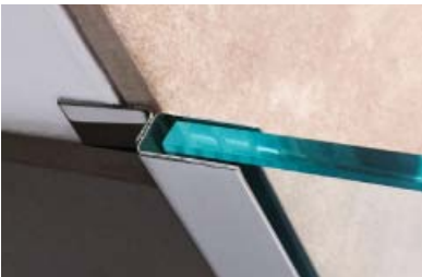
End “U” section Wall/Glass in “Linear”
