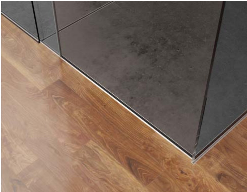
Shower entrance with 5 mm satin finish stainless steel threshold.
